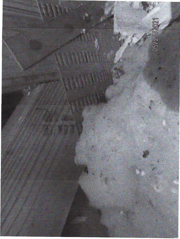
Metal Connector with 3 Nails on the Front Side & 0 Nails on the Opposing Side
