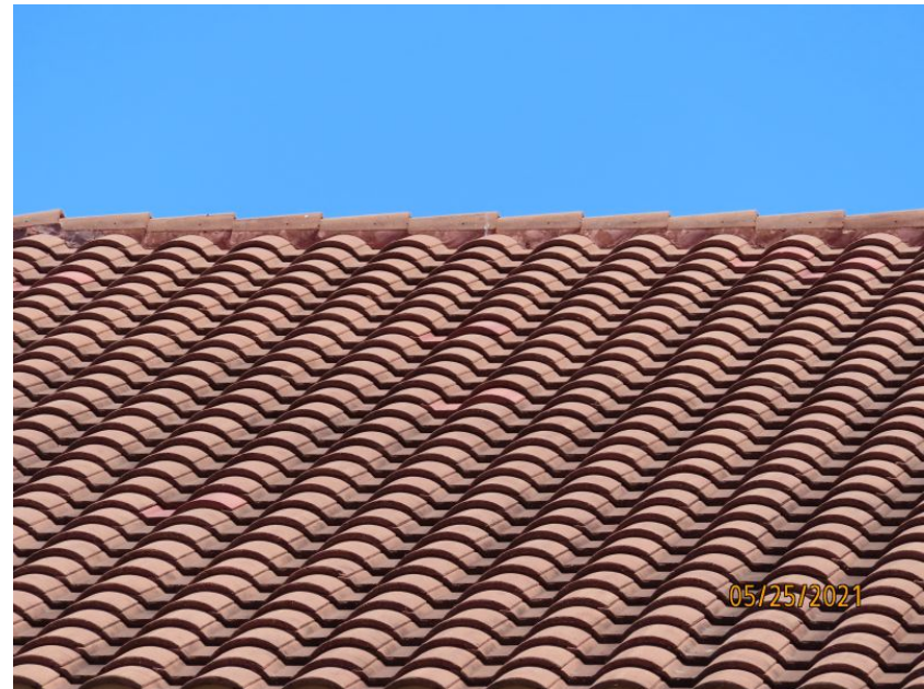
Concrete/Clay Tile Roof Covering
