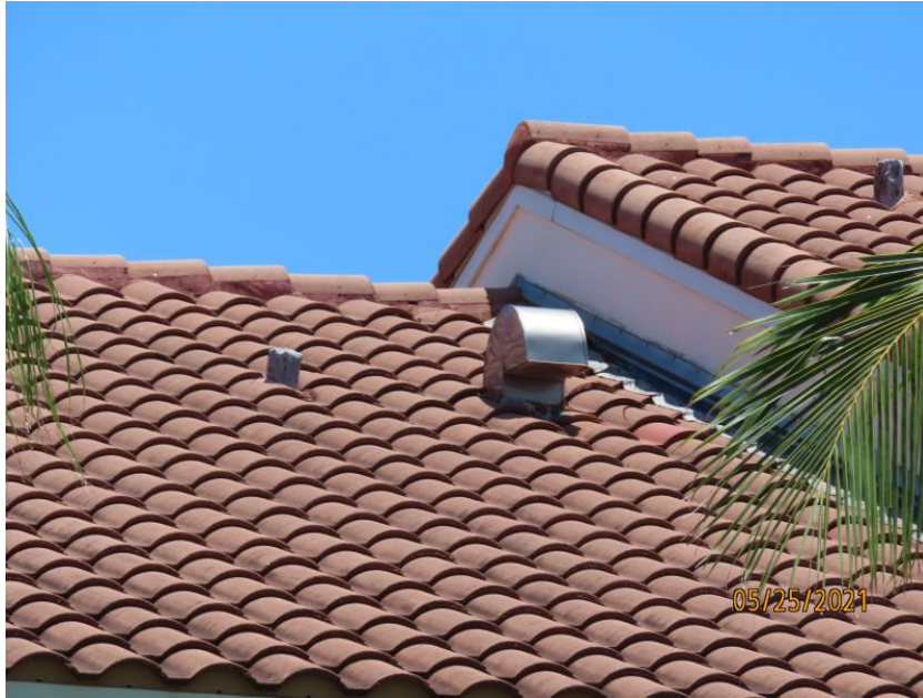
Concrete/Clay Tile Roof Covering
