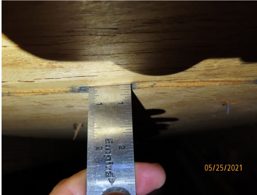
1/2" Deck Thickness Confirmed
