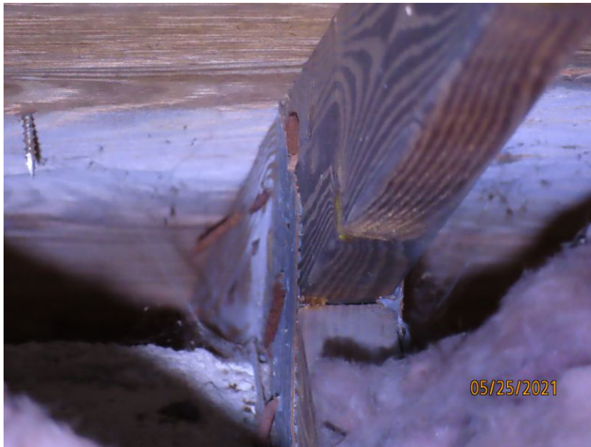
Metal Connector with 3 Nails on the Front Side & 0 Nails on the Opposing Side
