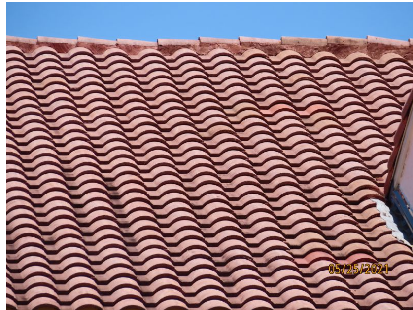
Concrete/Clay Tile Roof Covering
