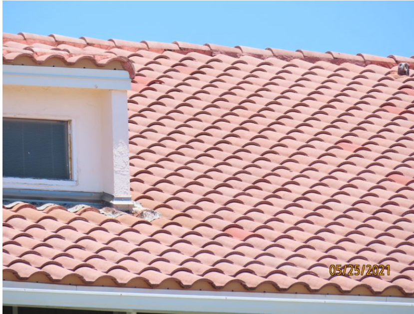
Concrete/Clay Tile Roof Covering
