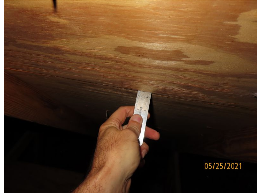
1/2" Deck Thickness Confirmed
