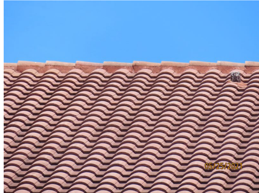
Concrete/Clay Tile Roof Covering
