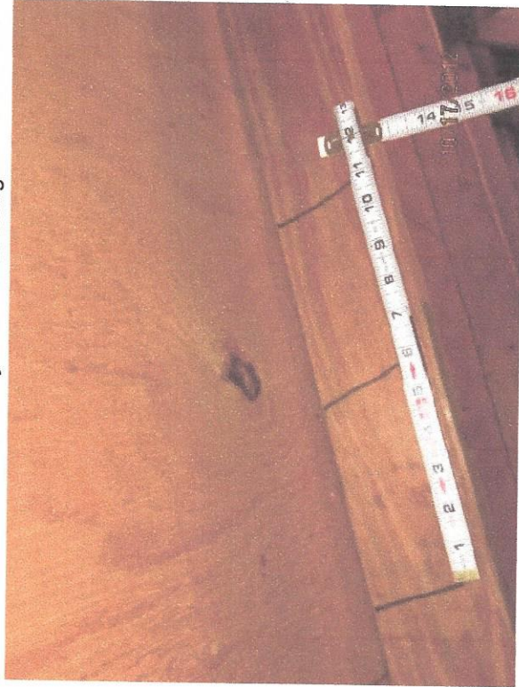
8d Nails Spaced 6" in the Field
