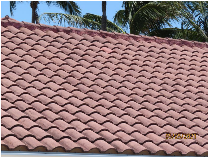
Concrete/Clay Tile Roof Covering
