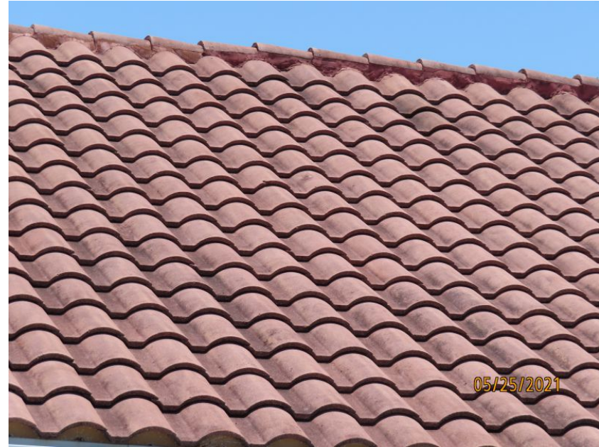
Concrete/Clay Tile Roof Covering
