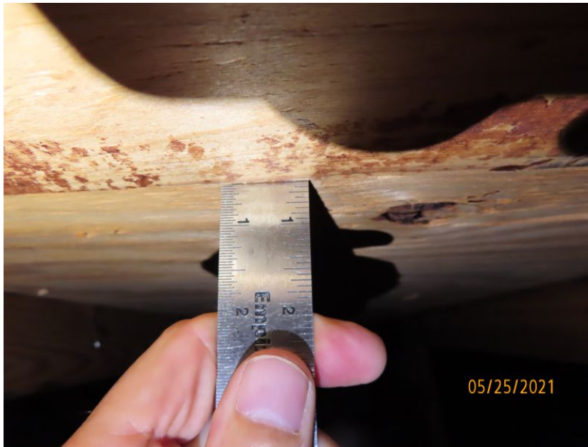
1/2" Deck Thickness Confirmed
