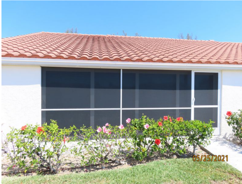
Unprotected Glazed Entry Door
