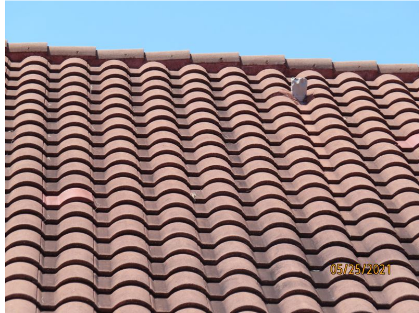
Concrete/Clay Tile Roof Covering
