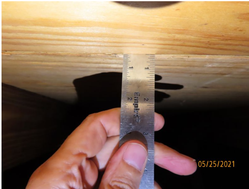
1/2" Deck Thickness Confirmed
