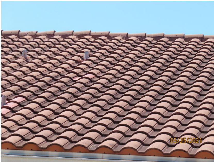
Concrete/Clay Tile Roof Covering
