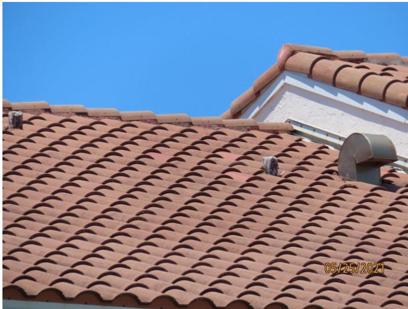
Concrete/Clay Tile Roof Covering
