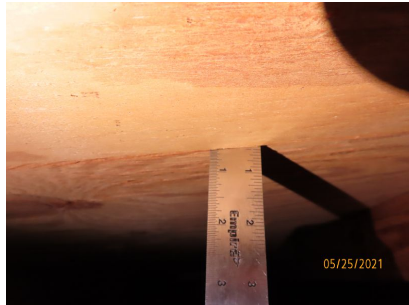
1/2" Deck Thickness Confirmed
