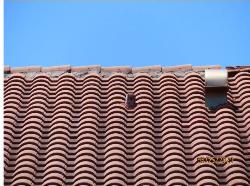
Concrete/Clay Tile Roof Covering
