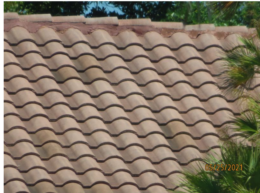
Concrete/Clay Tile Roof Covering
