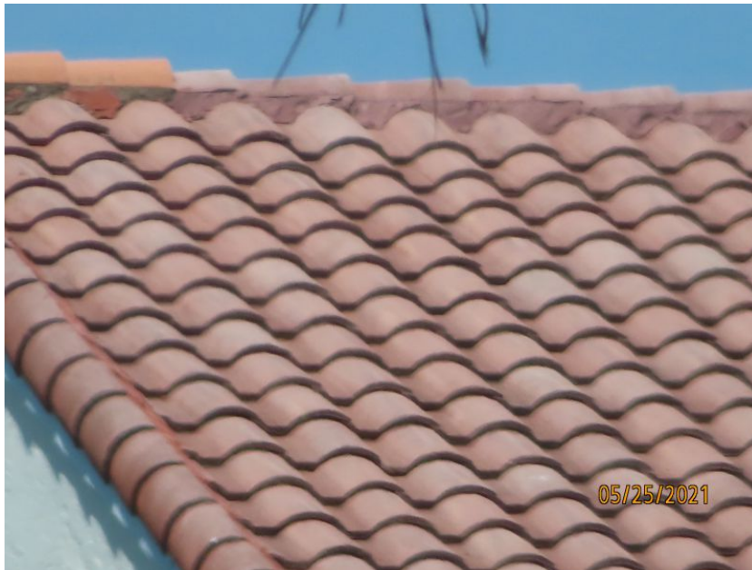
Concrete/Clay Tile Roof Covering
