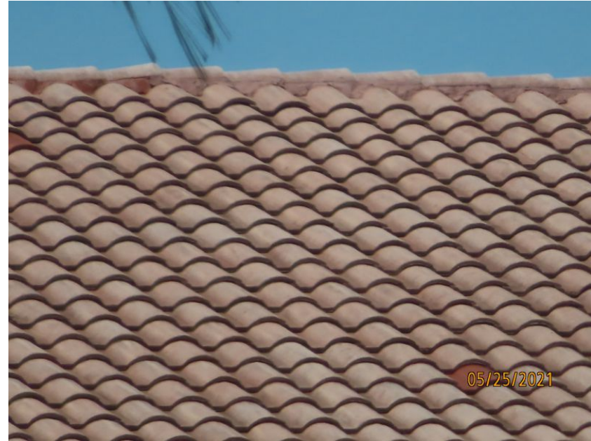
Concrete/Clay Tile Roof Covering
