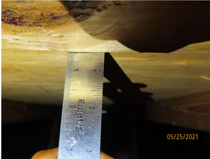
1/2" Deck Thickness Confirmed
